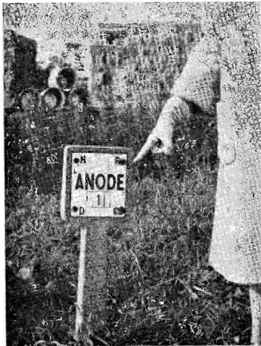
Always on the look-out for the odd picture or the unusual fact, this object protruding from the verge of a North Hertfordshire lane caught the attention of G5UM. On looking closer, Jack found that the sign also carried the legend "H.R.—D.C.," meaning nothing more exciting than Hitchin Rural District Council. As for that word "Anode," it is to indicate part of a system for the electrolytic protection of pipelines against corrosion! (We rely on Jack to keep us right up-to-date on such phenomena!)
